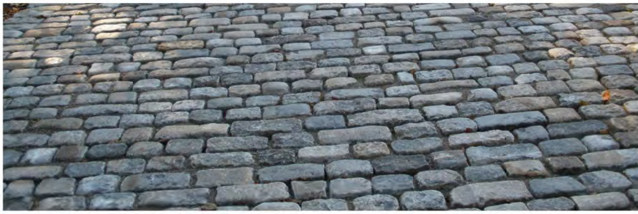
Granite Cobble Stone Apron on Driveway Entrance
