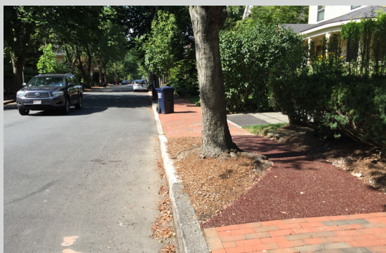
Final flexi-pave installation is being completed.
