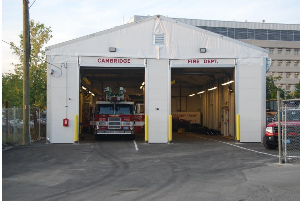
Temporary Fire Station at Smith Place
