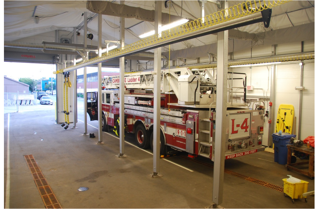
Interior of Temporary Apparatus Bay
