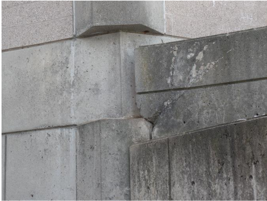
Photo 17: Expansion Joint South of the Gymnasium
