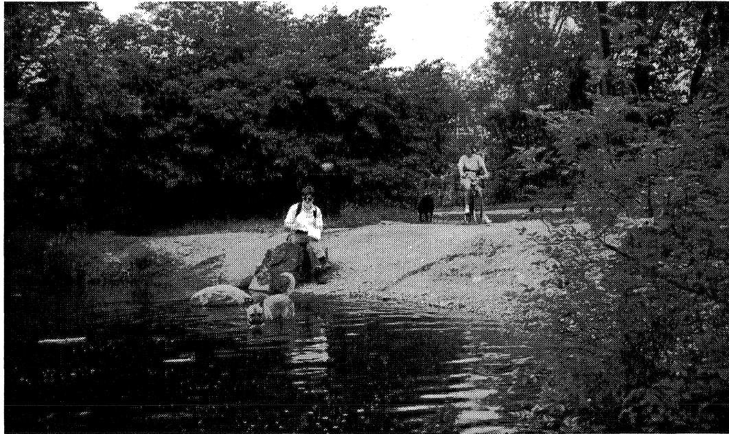
Figure 13: Bank Erosion along Little Fresh Pond, 1998 Source: Rizzo Associates, Inc., Summer 1998
