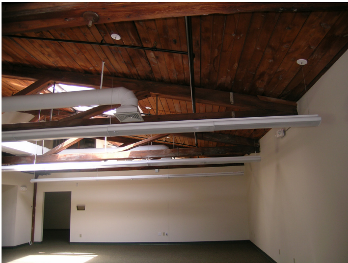
Current Foundry - view of South wing bay
