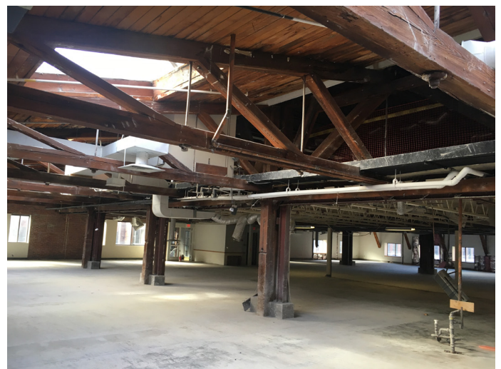
Current Foundry - third floor with exposed heavy timber trusses
