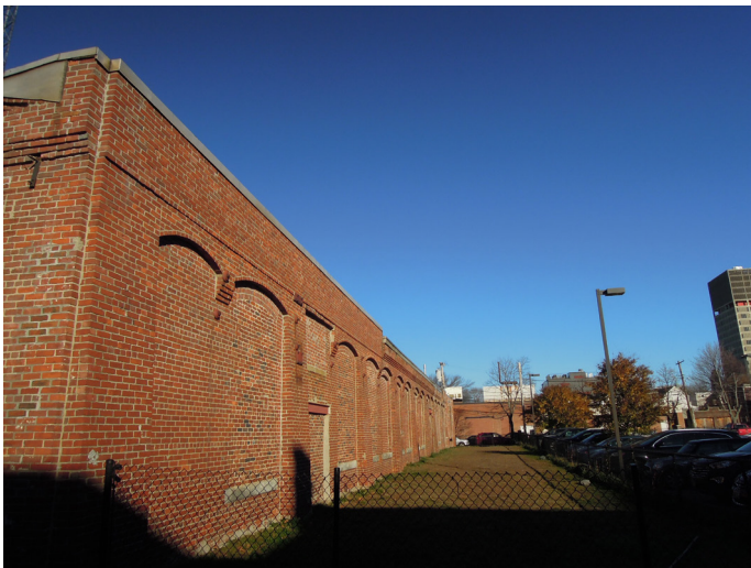
Current Foundry - view of outdoor space on South side
