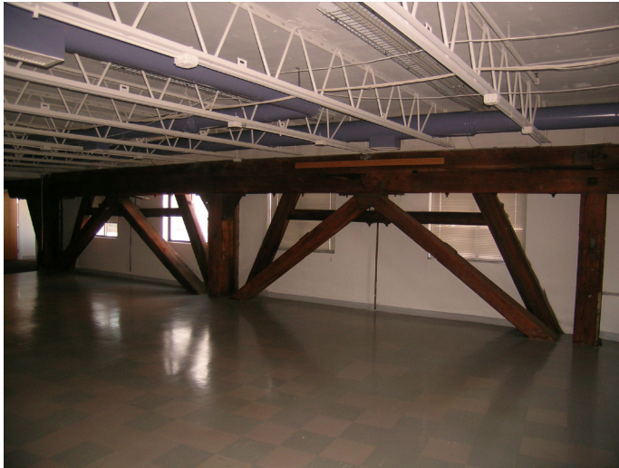
Current Foundry - view of second floor level
