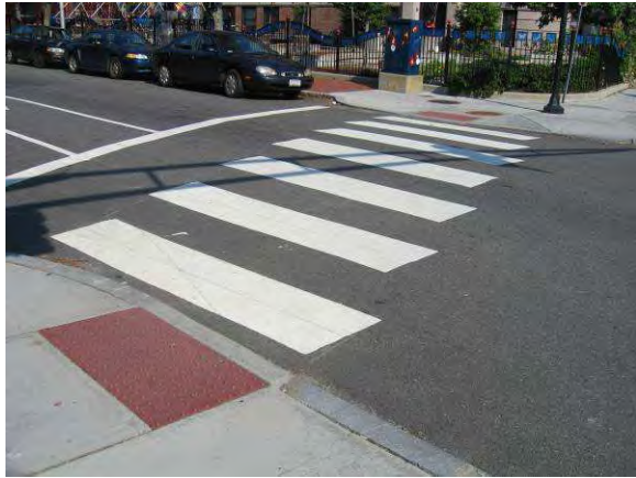
New crosswalk connecting parks and sidewalk repairs
