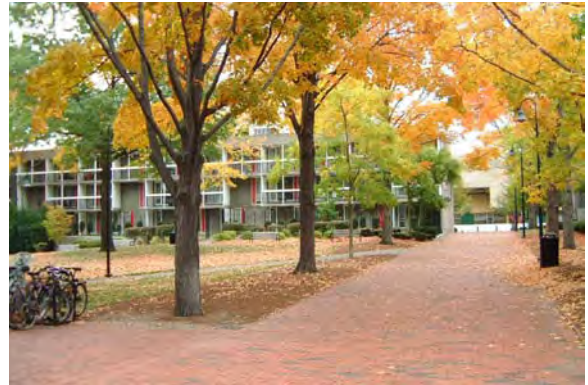
Figure 2.16 Peabody Terrace Courtyard
