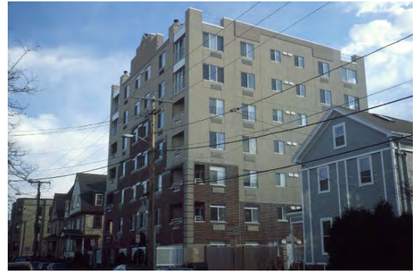
Figure 1.2 High-rise apartment house on Franklin Street
