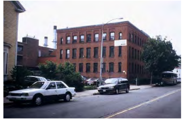
Figure 1.24 Office building on Putnam Avenue
