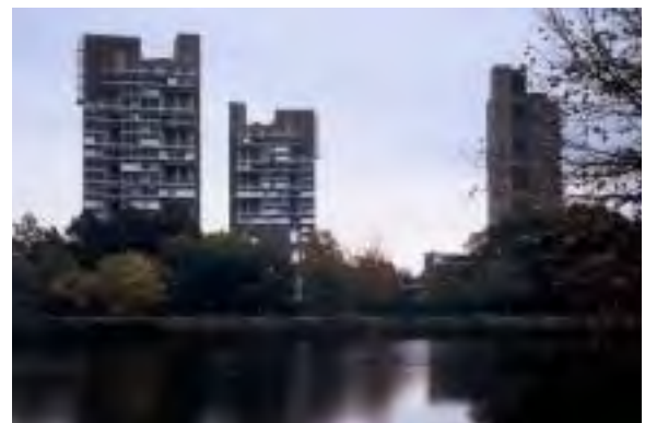
Figure A.3 Peabody Terrace
