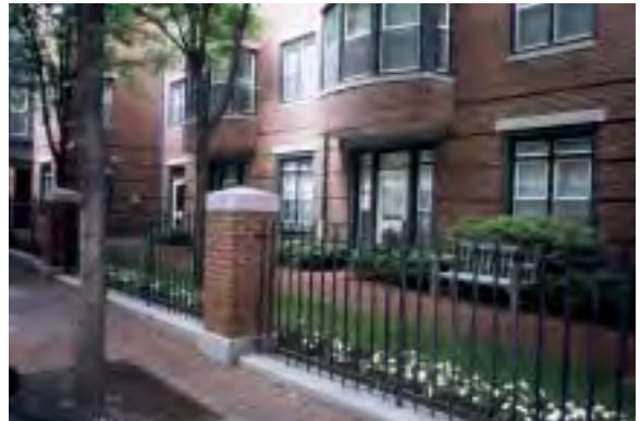
Figure A.4 Dewolfe Street Housing
