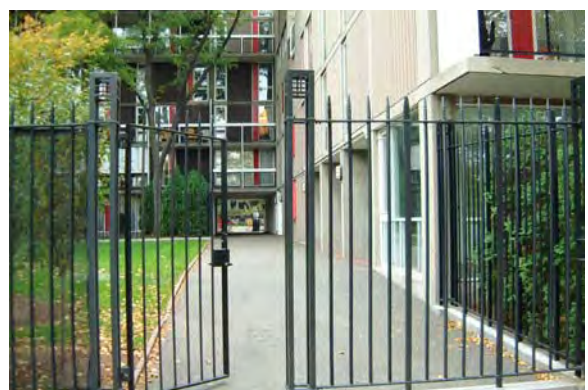
Figure 2.17 Fence at Peabody Terrace
