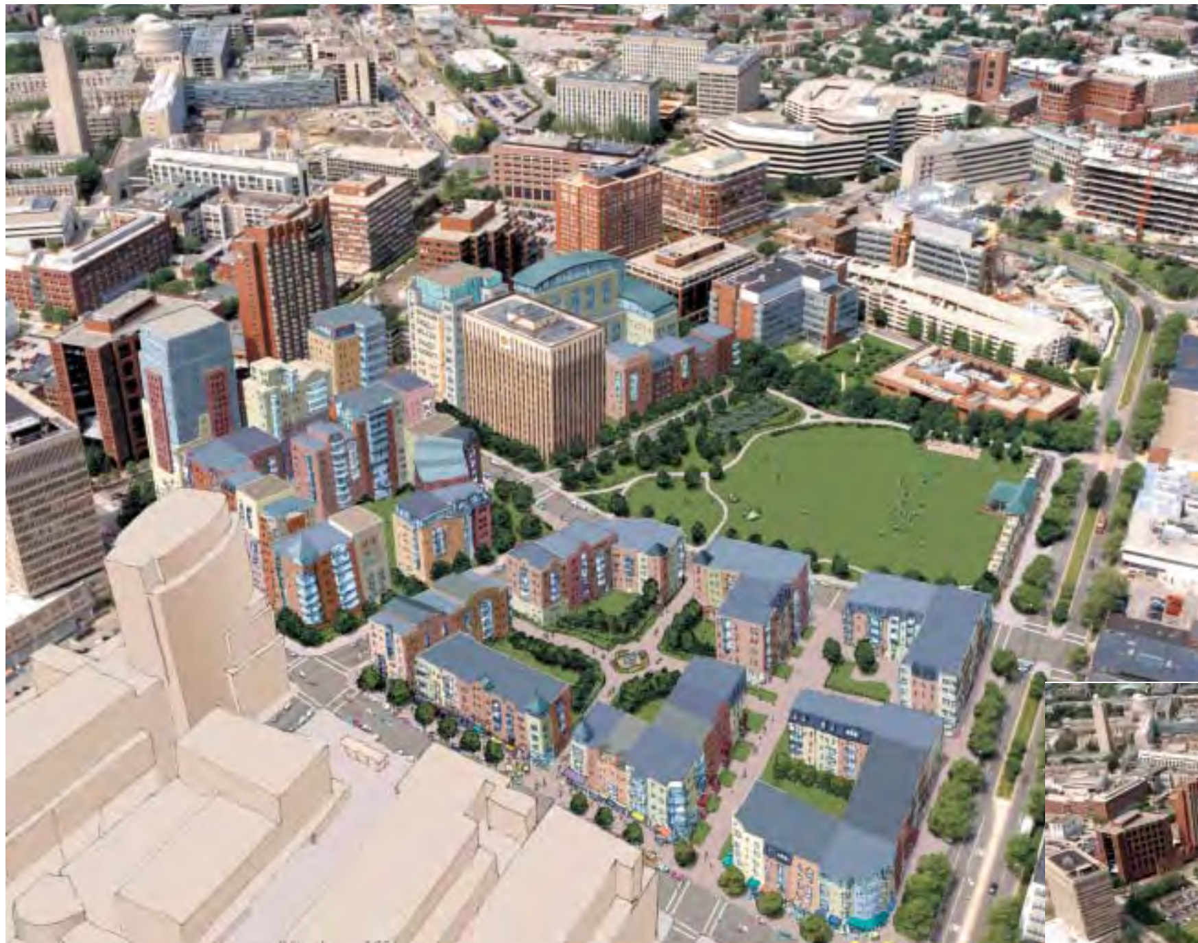
Illustrative study shows variety of blocks, transition in height, enlivened Third Street, and large neighborhood park. The park should be inviting and accessible to the existing residential neighborhoods and transition areas.
