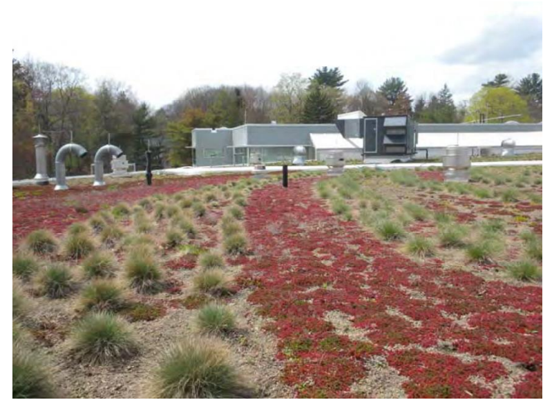
Green roofs on all flat roof buildings
