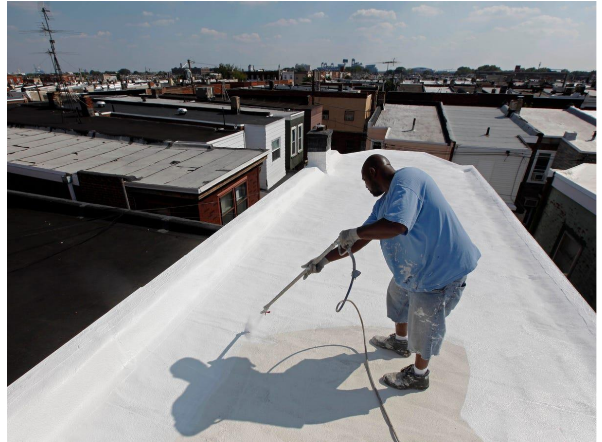
White Roof installation in New York City | Source: Business Insider
